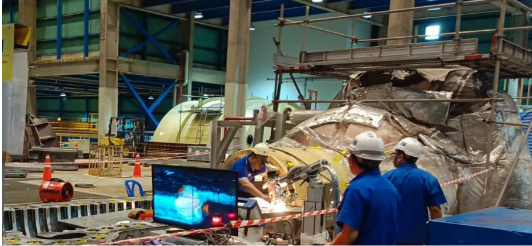
Fig. 13. Steam turbine casing repair using laser welding
